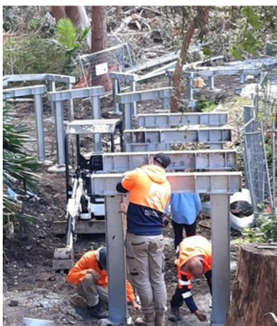
Walkway project: Top – pumping concrete for the footings to anchor the structure; a later concrete pour. Bottom – assembling the steel supports; Anthony Whitney removing some of the tree debris following the July storm and trees cleared for the project.
